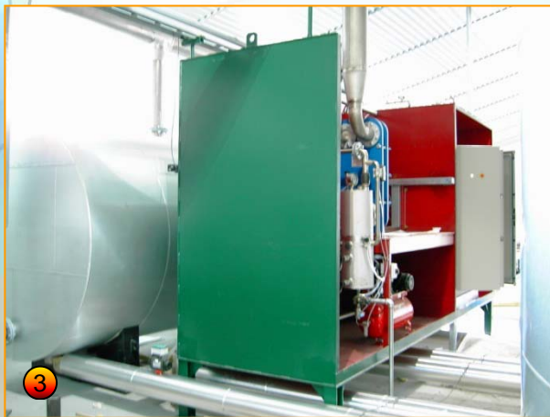
3-5: Compact equipment platform for the complete pump and valve unit, incl. of the electrical cabinet
